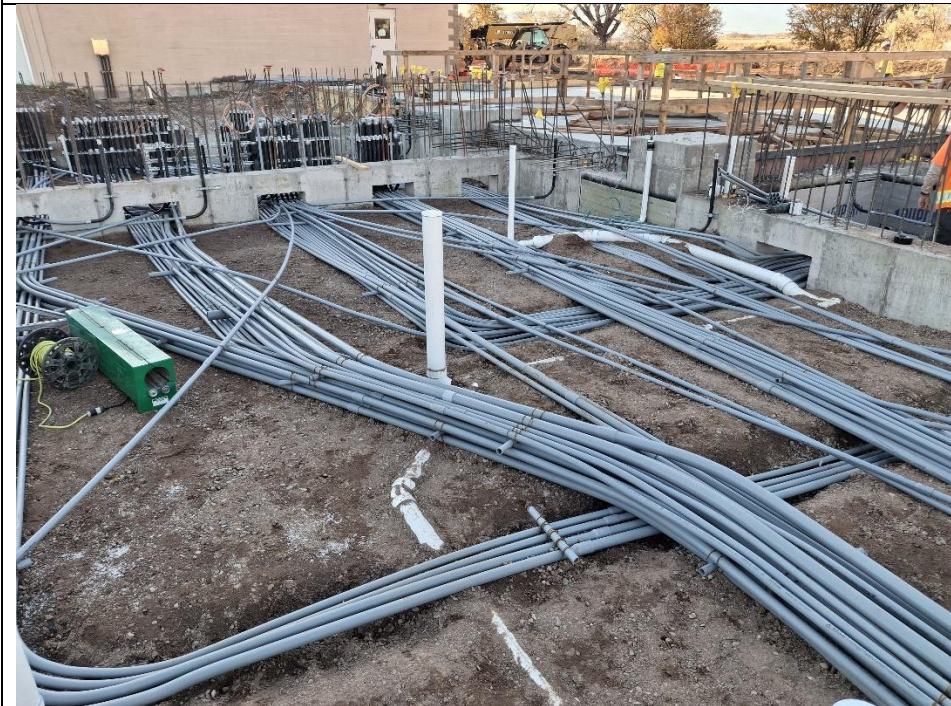
Continuation of Underslab Electrical Conduit
