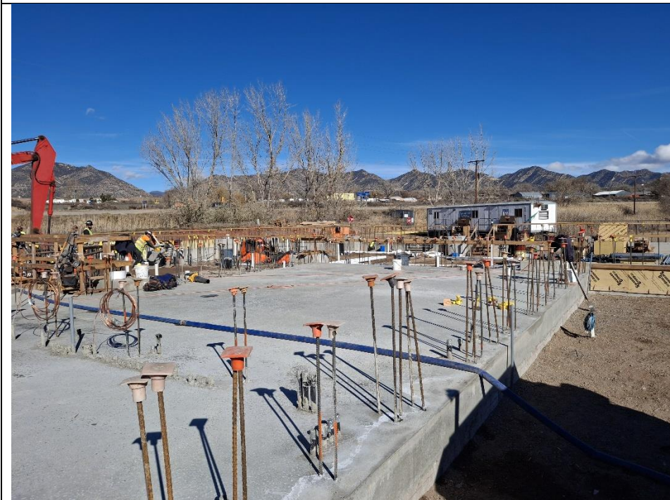
Electrical & Breakroom Slab- on-Grade Concrete II
