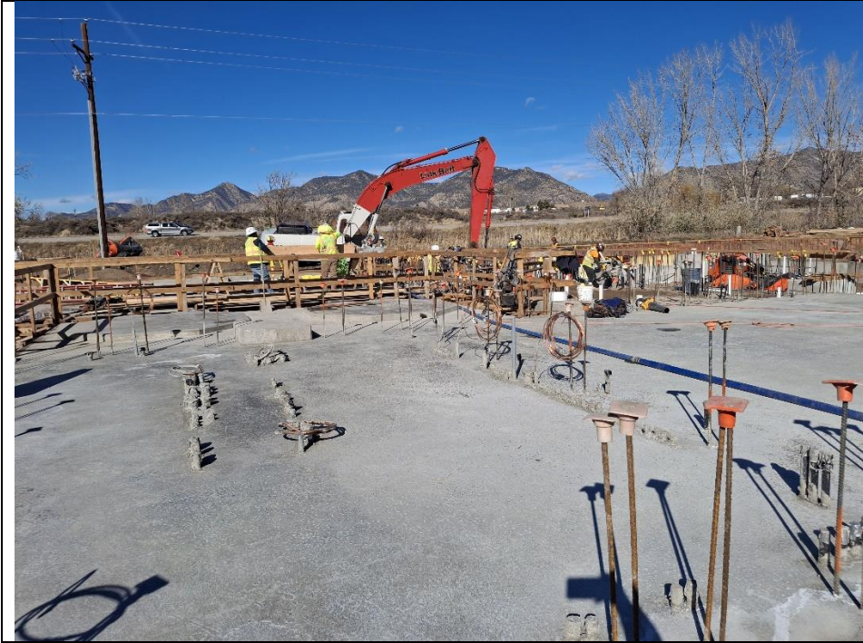
Electrical & Breakroom Slab- on-Grade Concrete
